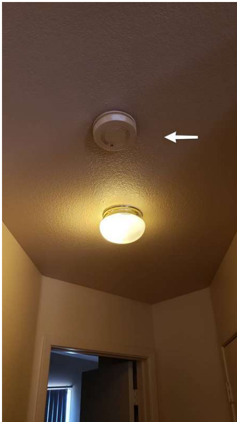
Hallway - 2nd Floor
