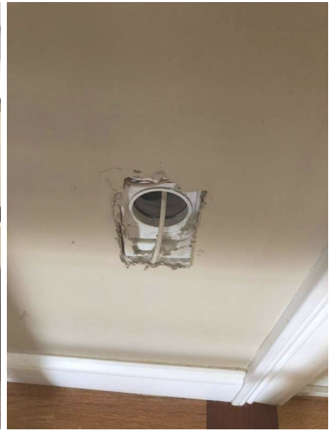
Main floor entry way. Missing cover plate.
