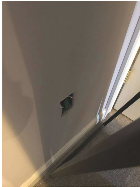
2nd Floor hallway missing cover plate. 2nd Floor bedroom. Missing cover plate.
