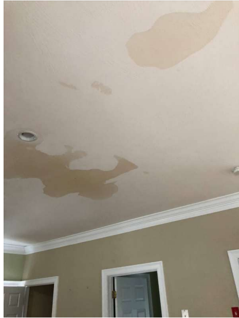
Moisture stains in kitchen ceiling tested negative for moisture at time of inspection.
