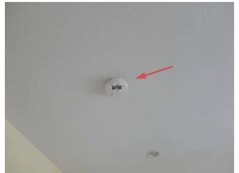
Smoke alarm in 2nd floor north bedroom missing battery.
