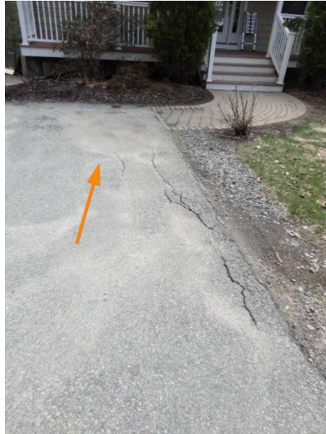
Uneven pavement may cause a safety issue during winter months (ice hazard).
