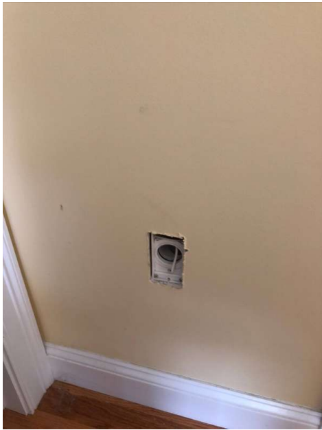
2nd Floor hallway missing cover plate. 2nd Floor bedroom. Missing cover plate.
