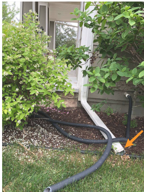
Repair - Recommend that extensions carry water out 4-6 feet from the house.
