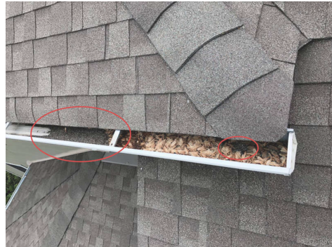
Significant aggregate washed off the shingles.
