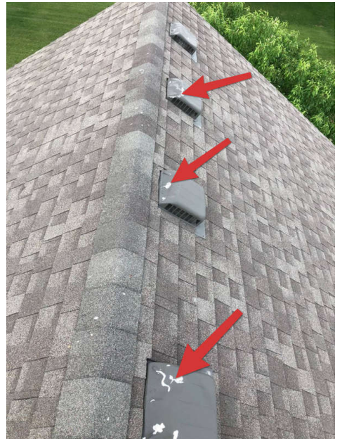
Damage on the vents.
