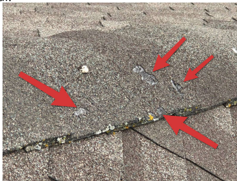
Fiberglass mat exposed by damage.
