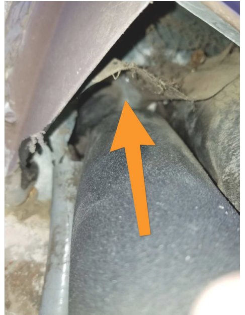
AC Lines South Exterior
