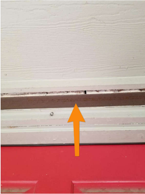
Above Front Door
