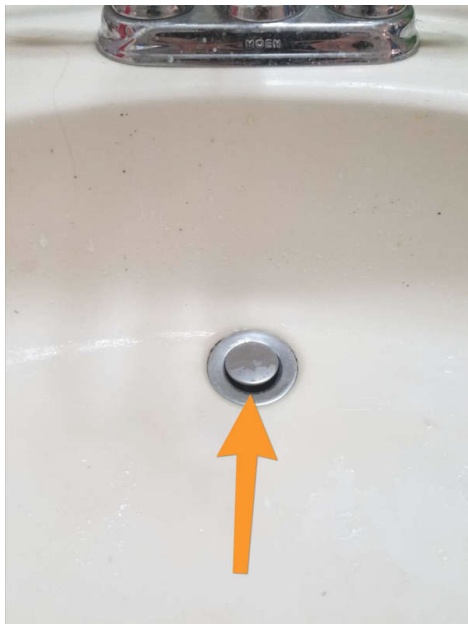
2nd Floor Bathroom
