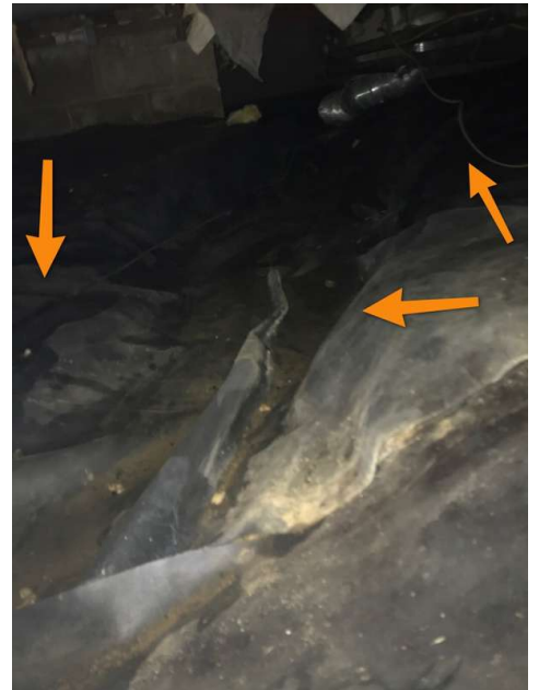
Standing Water In Crawlspace
