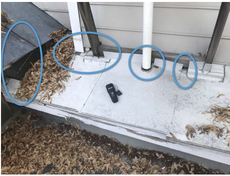
Improper Flashing
