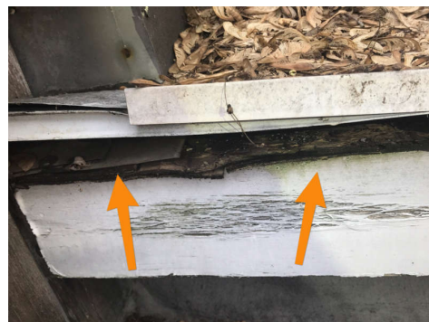
Deteriorated Roof Sheathing
