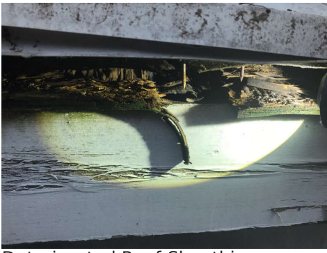
Deteriorated Roof Sheathing
