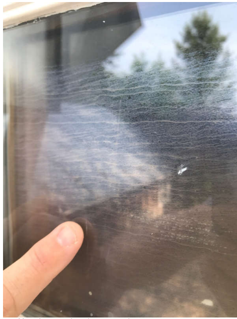
Failed Seal Close View
