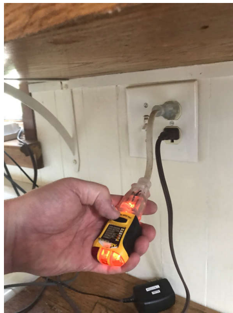
No GFCI In Kitchen (Near Sink)
