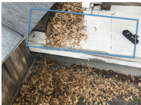
Moisture Intrusion / Deterioration of Wood Sheathing Beneath Flashing
