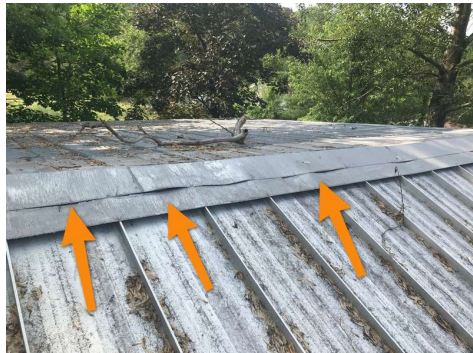
Unsealed Areas Of Ridge Vent
