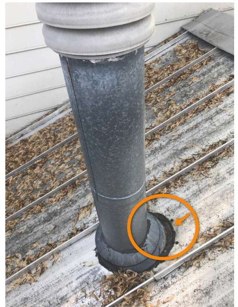
Roof Sealant Traps Water
