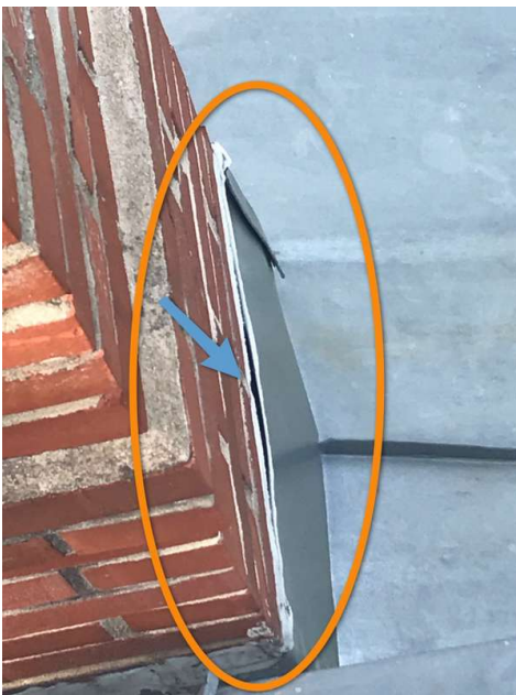
Chimney Flashing Separated From Masonry
