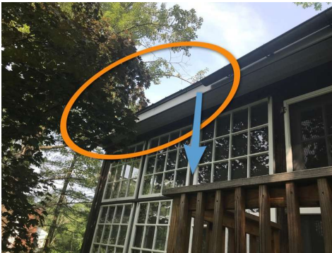
Missing Gutter And Downspout
