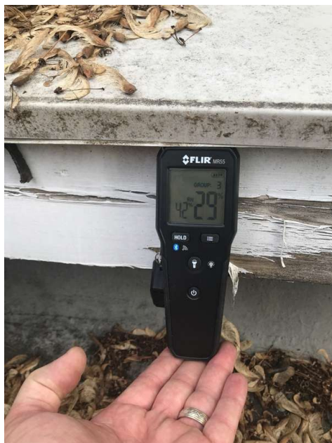
Elevated Moisture Level In Wood Sheathing
