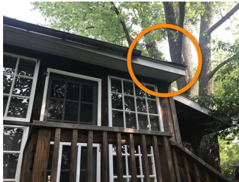
Missing Gutter
