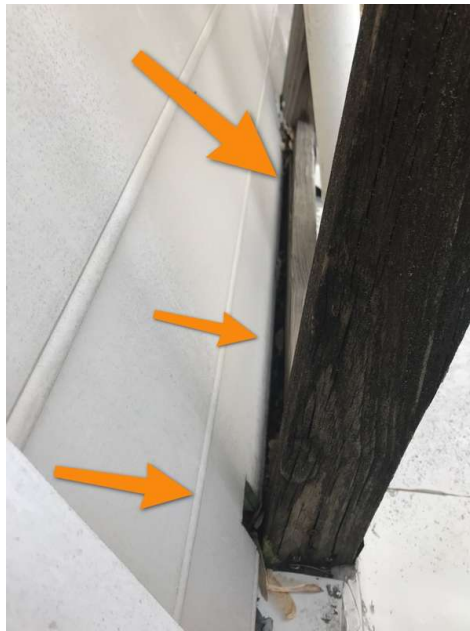
Missing Flashing / Unsealed Penetrations
