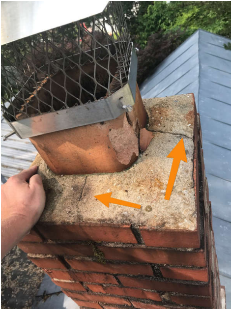
Cracked Chimney Crown
