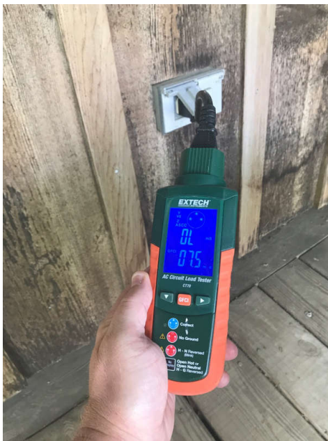
No GFCI On Front Porch
