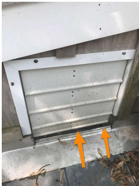
Gap In Flashing Below Sunroom Vent Fan
