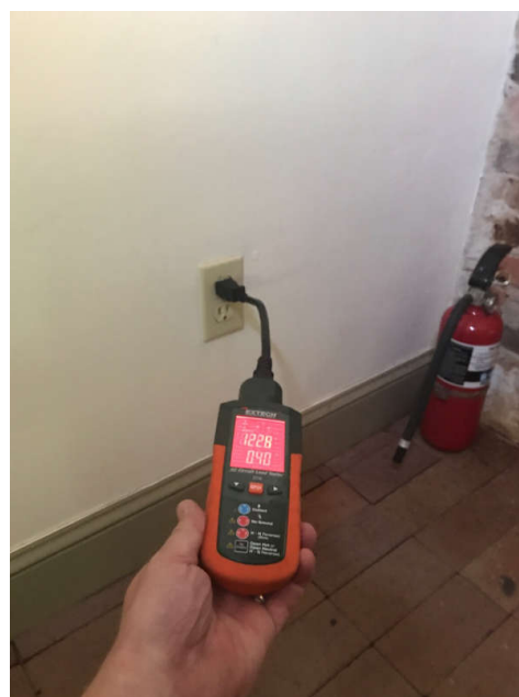
Ungrounded Receptacle (Behind Wood Stove)
