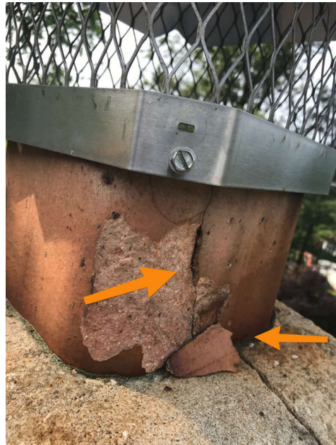
Cracked Chimney Flue
