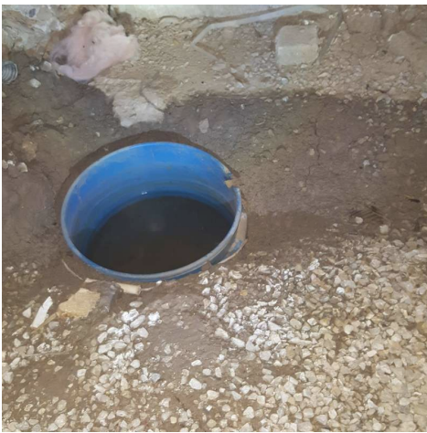
Bucket, full of water, buried in trench in the addition crawl by the sump pit
