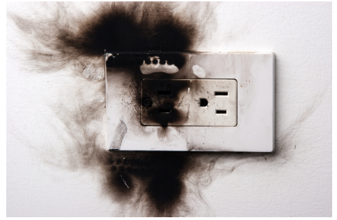
Scorch marks on cover plate
