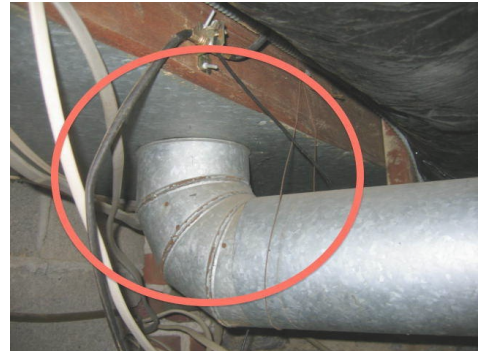
Loose connection; recommend sealing.
