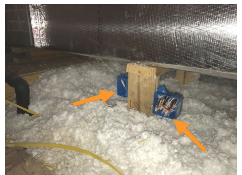
Attic Under AC Cabinet Plenum
