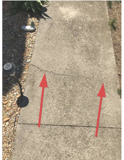
Minor walkway crack.
