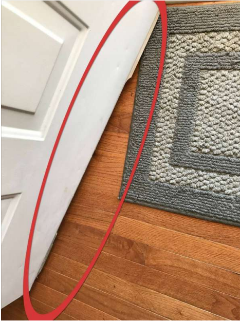
Front door. Damaged weatherstripping along bottom of door.
