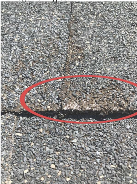
Damaged shingles.
