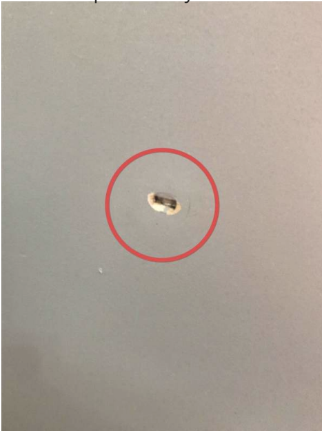
Doorknob hole, living room front door.
