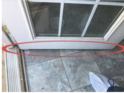
Front door. Damaged weatherstripping along bottom of door.
