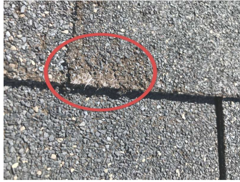
Damaged shingles.
