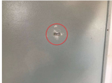
Doorknob hole, kitchen basement door.
