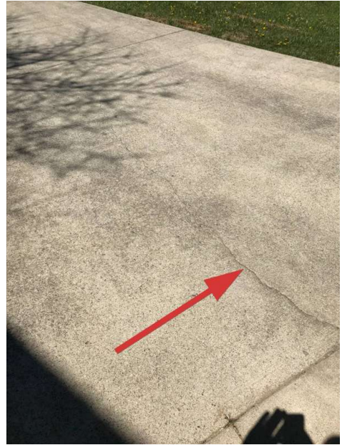
Minor driveway crack.
