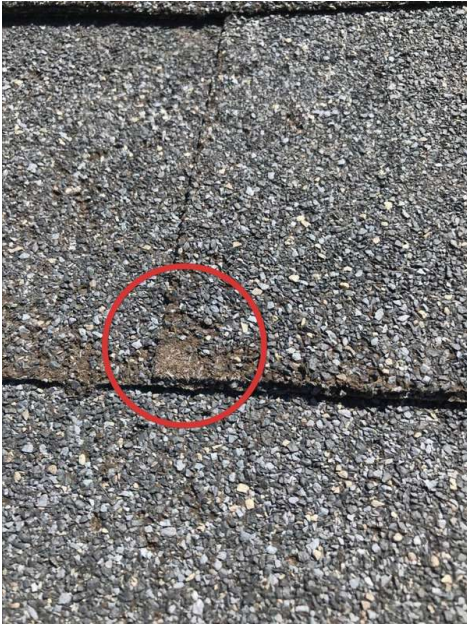
Damaged shingles.
