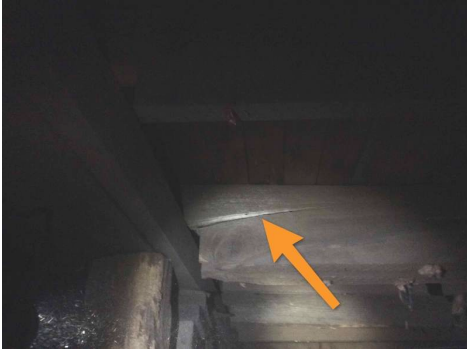
Joist has cracked
