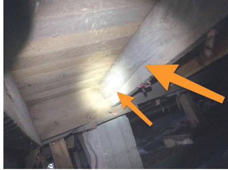
Joist have cracked
