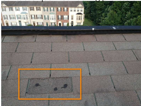
Missing Shingle (Rear Side of Roof)
