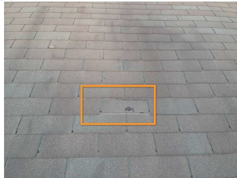
Missing Shingle (Front Side of Roof)
