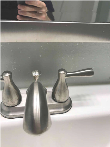
Water spray from faucet not having water control device at tip
