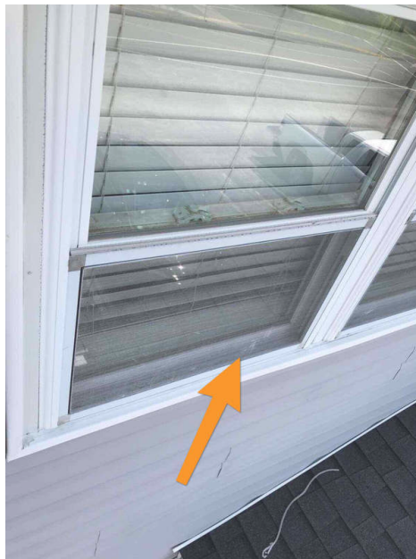
Window Screen showed minor holes from wear
