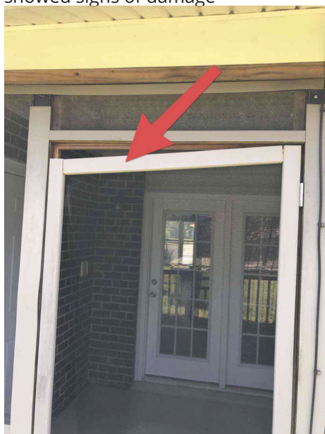
Screen Porch Door had Large Gaps and was not sized properly
