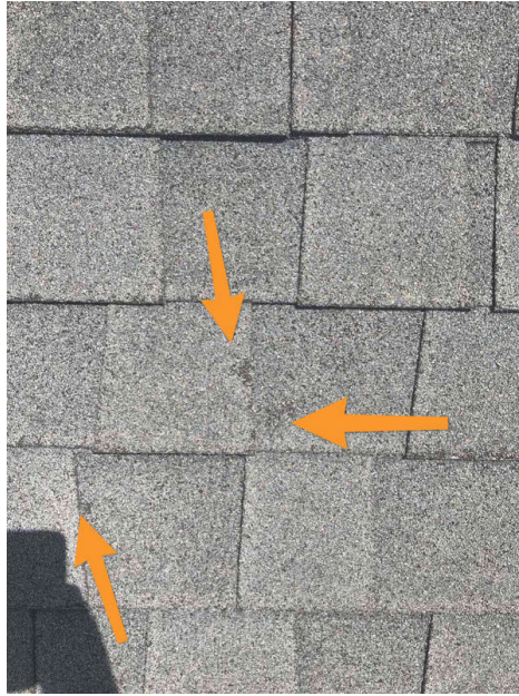
Small blisters and granule loss.
