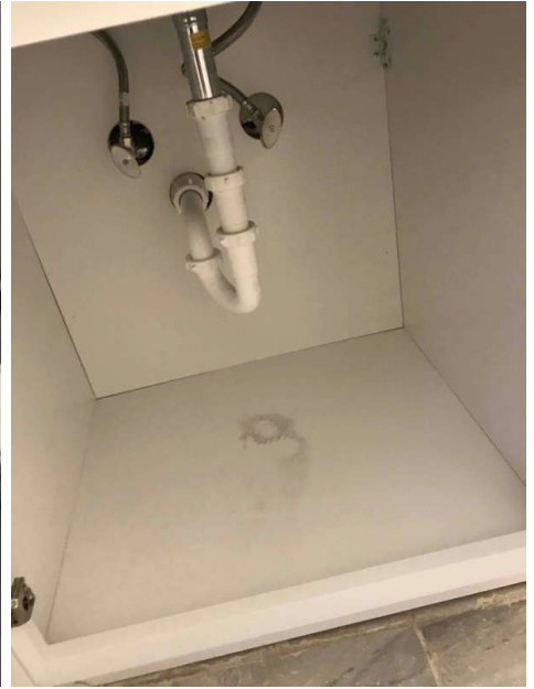
P-trap leaking downstairs / area was dry so may be old
