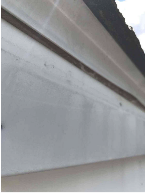
Exposed wood under drip edge
