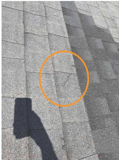
Shingles cracked from repair
