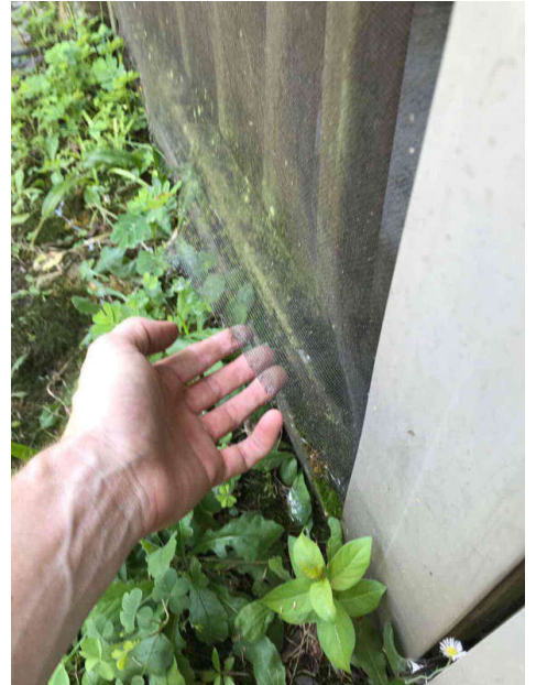
Damage along Bottom Edge of Screen on Porch
