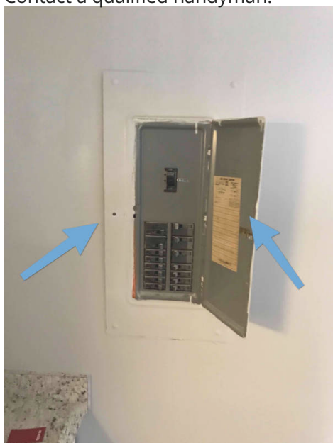
Panel Screws Missing on both Sides
