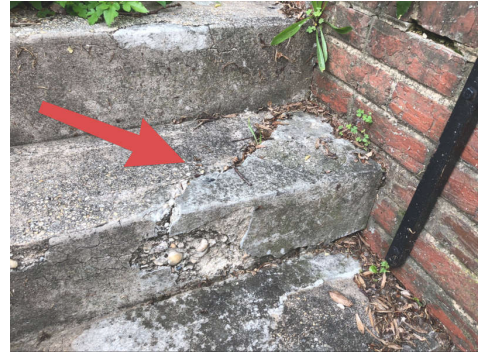
The cracked section of concrete is starting to come loose
