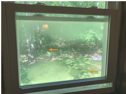
Crack in window. Failed seal
