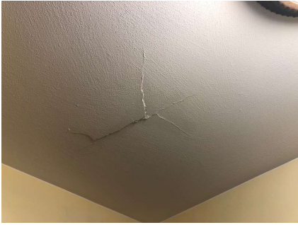
Crack in hallway. 2nd Floor
