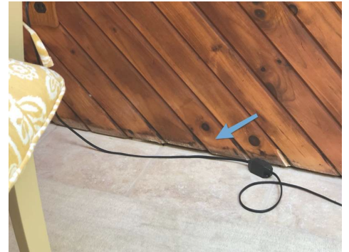
Floor to wall connection. Sunroom
