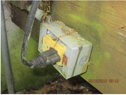
GFCI not protected with weather-proof cover. Not tested.
