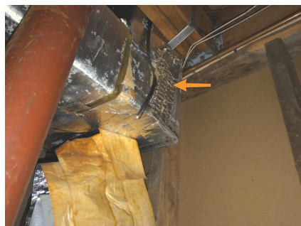
Insulation loose and falling off distribution ducts.
