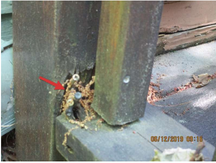
Railing damaged and loose.
