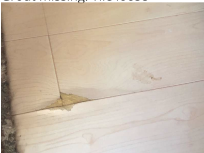
Dining Room. Floor damaged.
