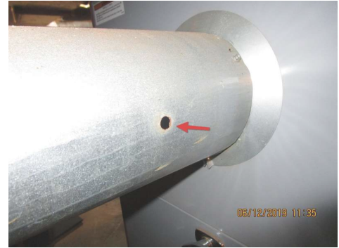
hole in flue vent pipe
