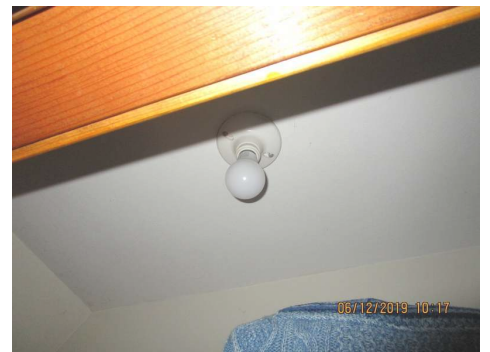
Improper and no switch located
