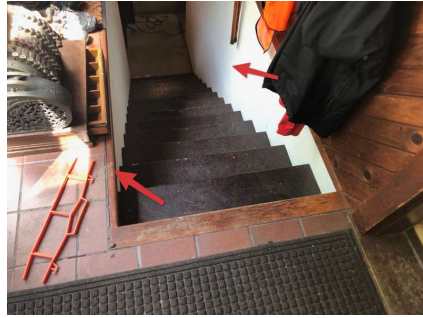
Missing railings and graspable handrails.
