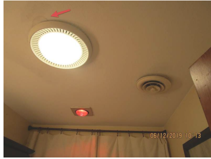
Stain observed in bathroom. 2nd Floor
