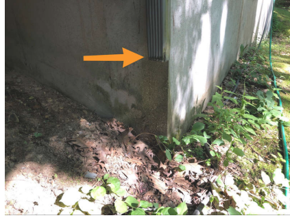
Downspout extension needed
