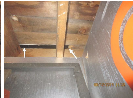
Sliding door. Basement view
