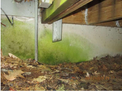
Downspout extension needed
