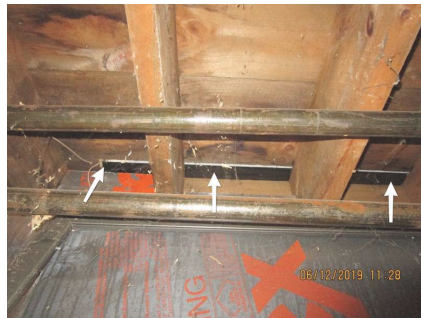
Sliding door. Basement view
