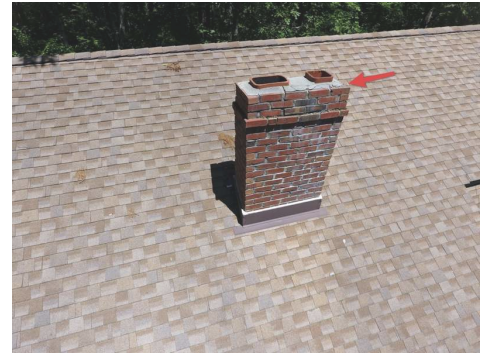
Chimney crown. Cracked mortar
