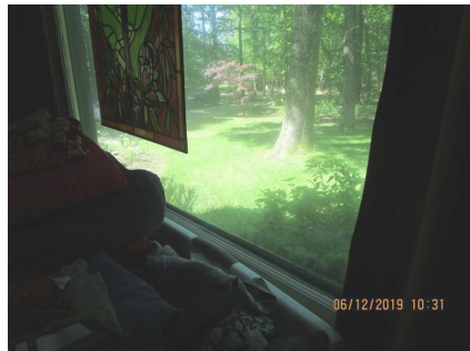
Failed Seal. Living Room
