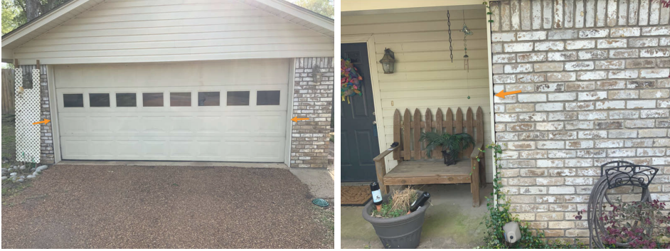
Right side of front porch
