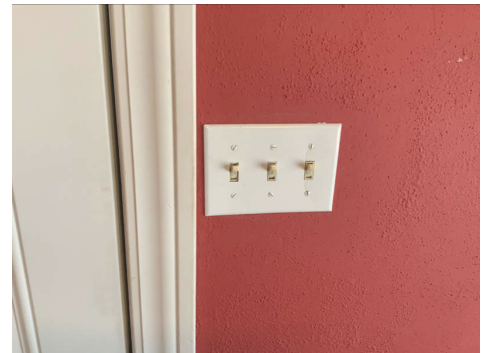
Next to garage door
