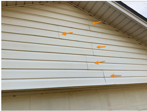
Over garage door
