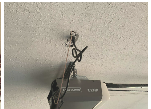
Garage door opener receptacle.
