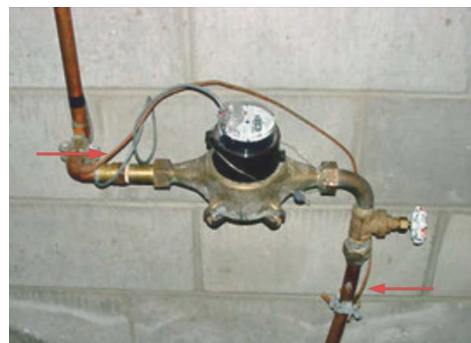
Example of a bonding jumper at the water meter
