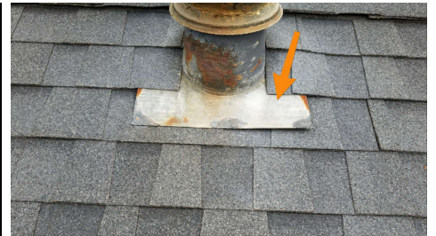
Loose, nail heads exposed
