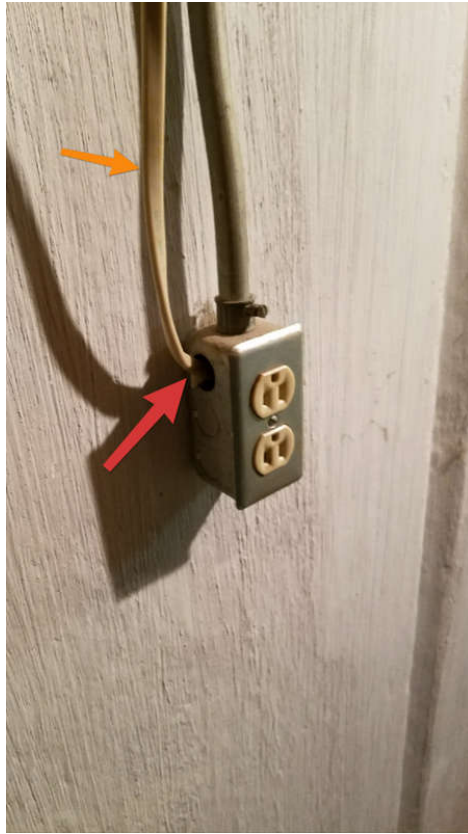
Also note missing cable clamp
