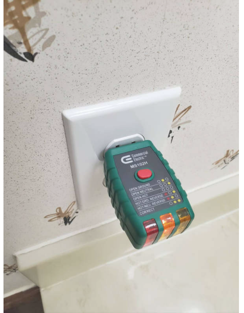
Hallway bathroom - left of sink
