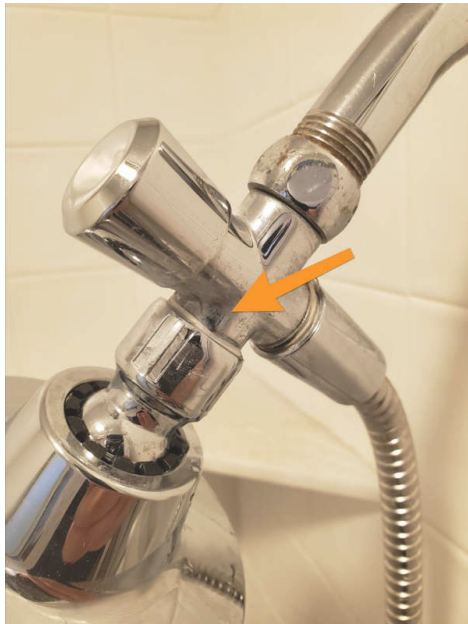
Leak at fitting - master
