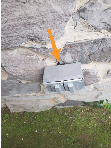
Front right side - loose and needs secured
