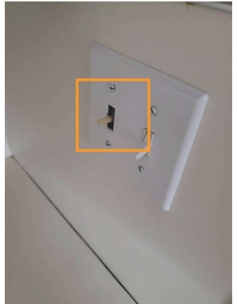
Control kitchen ceiling fan speed
