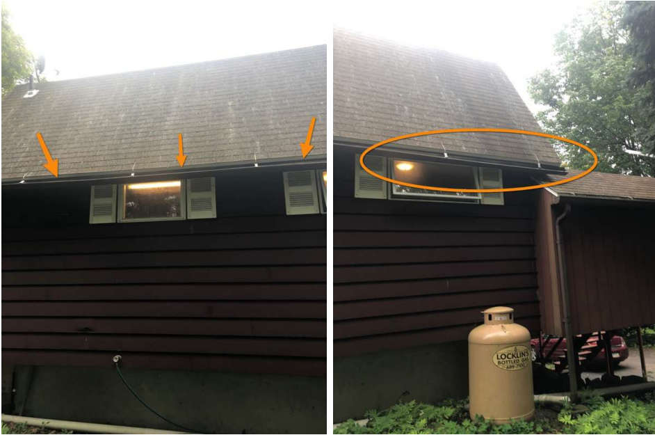
The gutter brackets may be reused. Although the gutter was observed to have twisted the brackets appeared to be intact.
