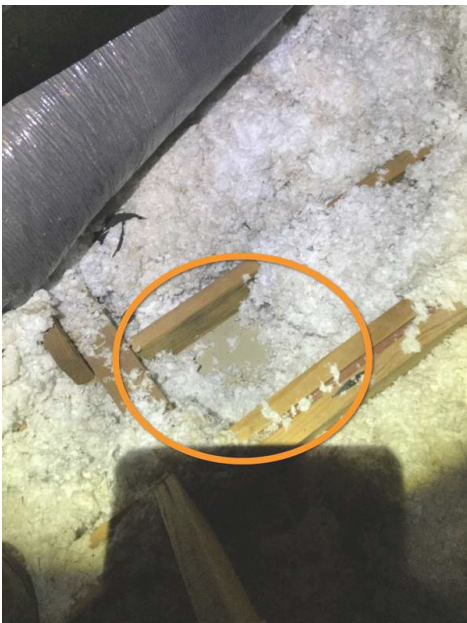
Above Laundry Room Hallway
