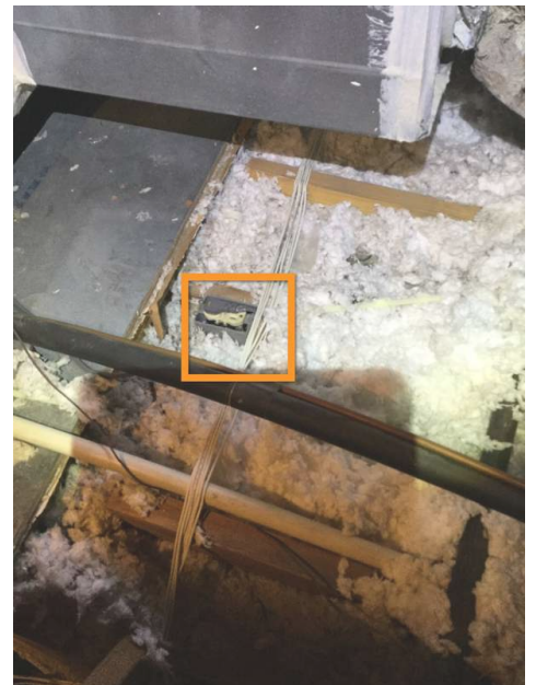
Front right of furnace
