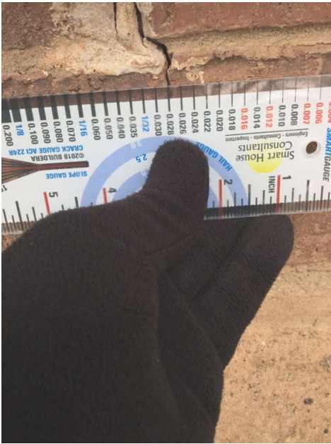
West Wall Close Up
