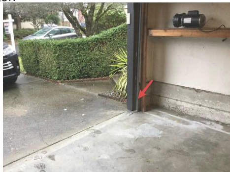
photo-electric sensor should be here.
