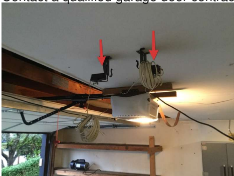
Photo-electric sensors are at ceiling. They should be at the door rail near the
