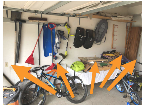
Five receptacles inoperable
