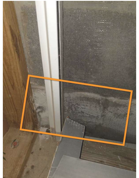
Basement Bedroom Closet
