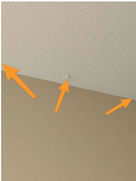
1st Floor Bathroom
