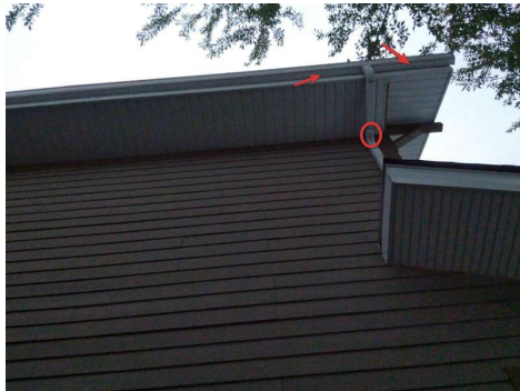
signs of over flow
