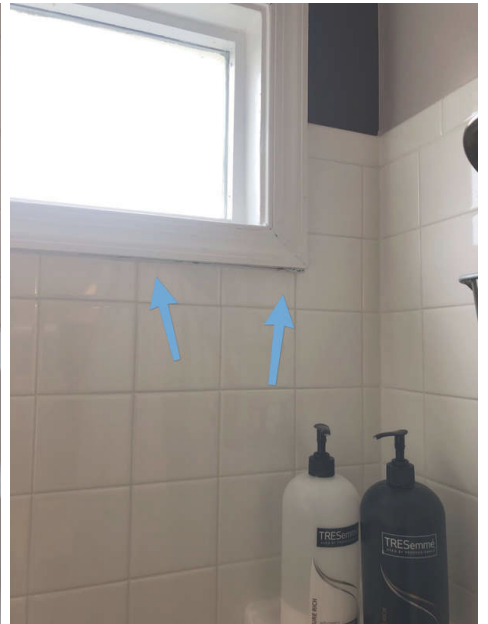
2nd floor Bathroom
