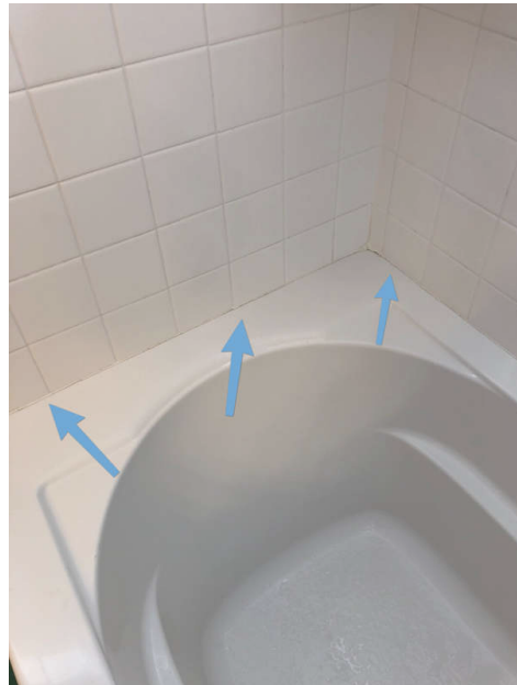
2nd floor Bathroom
