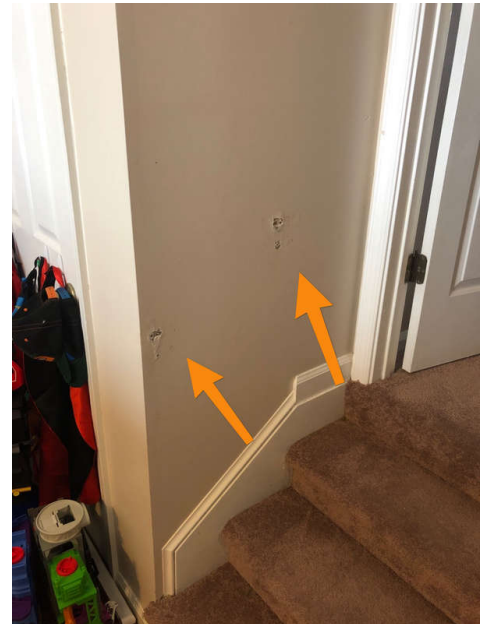
2nd floor above garage
