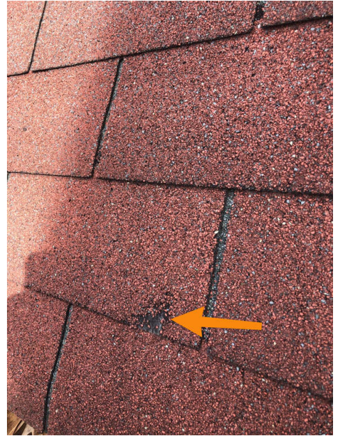
Rear garage near gutter edge
