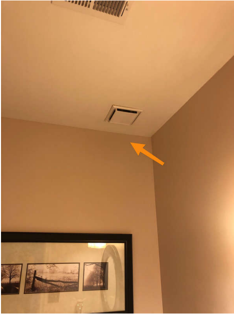
1st Floor Bathroom
