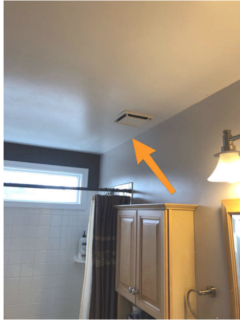
2nd floor Bathroom
