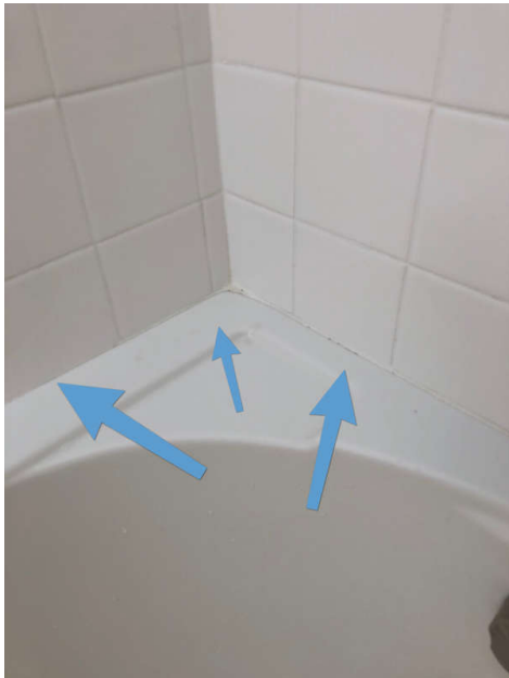
2nd floor Bathroom
