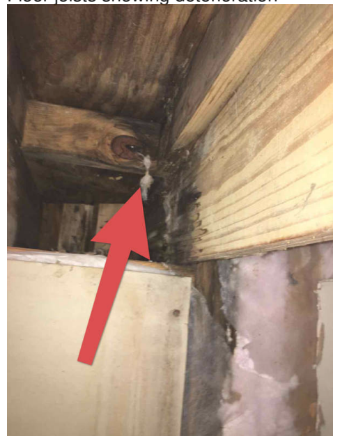
Floor joists showing deterioration
