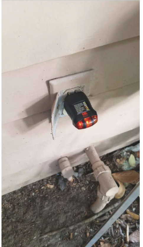
Front reverse polarity
