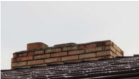
Cracked bricks
