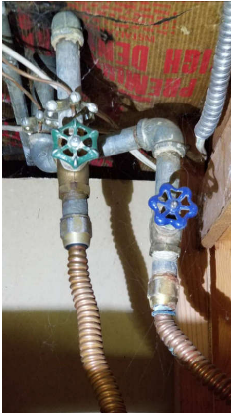
Basement water heater
