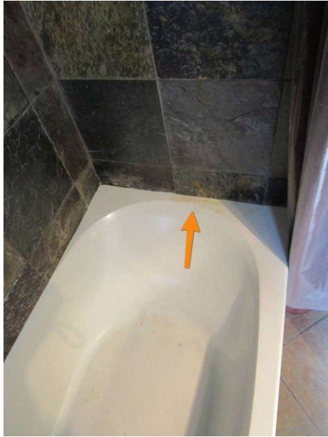
Some staining on master tub surface.
