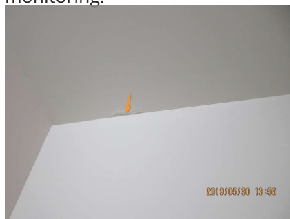
Joint tape starting to come undone. Recommend repairing.
