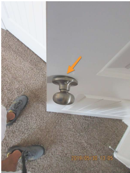
Top of laundry door. missing latch. Recommend replacing.
