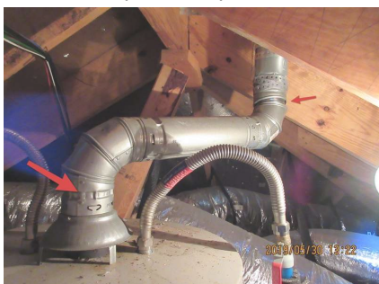
Exhaust should have a 12" minimum straight rise out of the water heater before a turn. broken exhaust flue.
