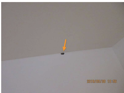
Hole in wall in alcove in garage. Recommend repairing
