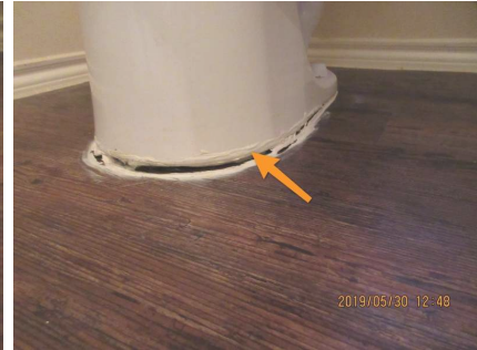
Recommend caulking around toilet. Toilet also appears to be lifted. This could be from using an incorrect toilet ring size. Recommend having a licensed plumber come out and evaluate.
