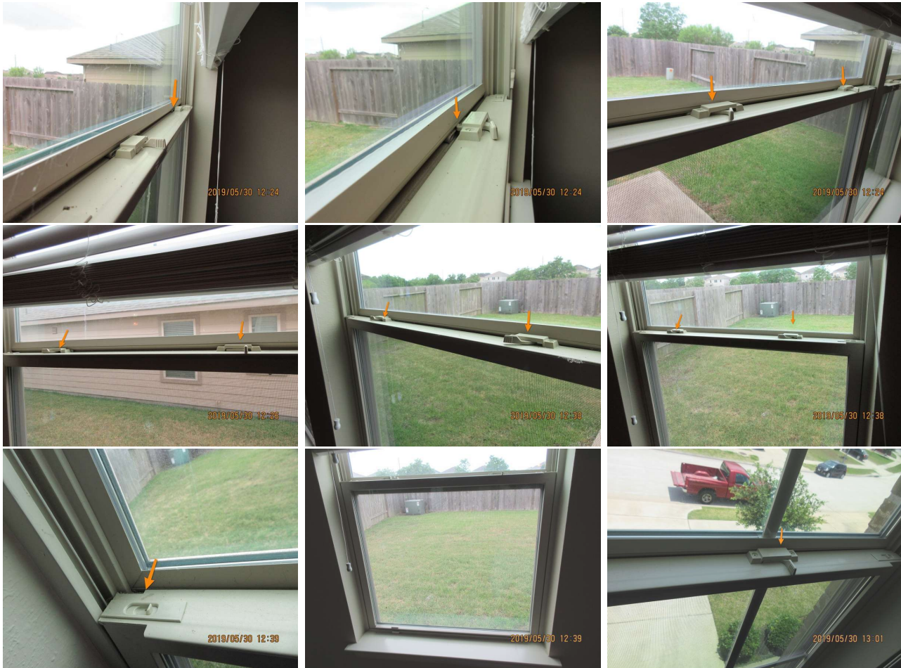
This window is off the railing.
