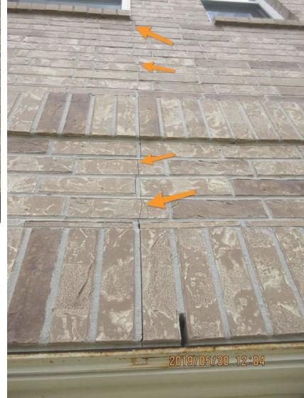
Cracked brick. See comments in "Foundations"
