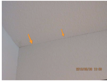
Crack starting to form on ceiling/wall joint. Recommend monitoring for future expansion of crack. This along with comments made in foundations section, recommend evaluation by structural engineer.
