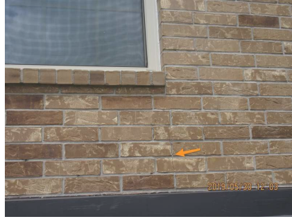
Cracked brick. See comments in "Foundations"
