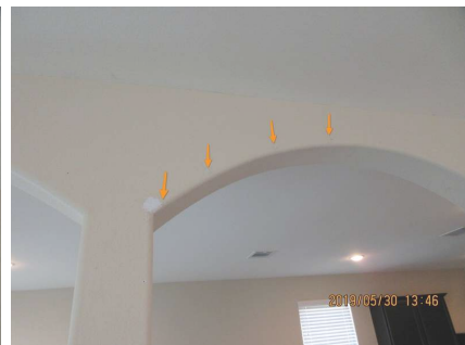
Repairs above arches. Recommend finishing repairs.
