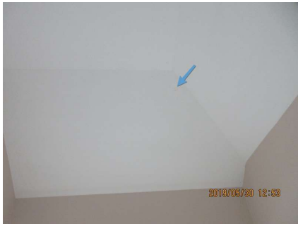
Previous repairs. Recommend asking what this was from.
