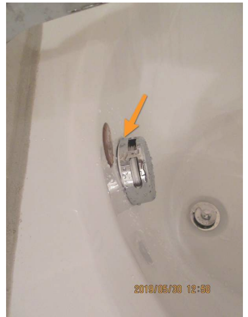
Recommend sealing around this as moisture can get behind and cause issues.
