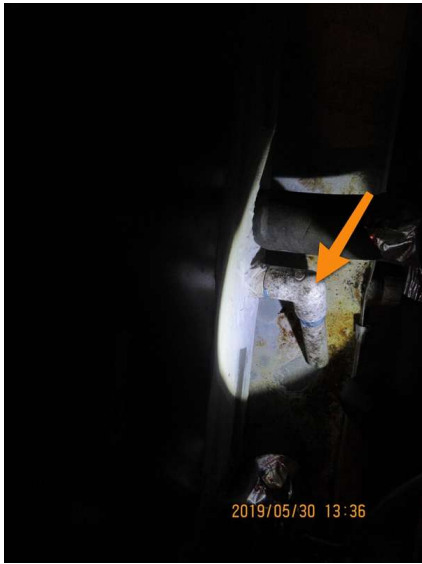
Organic growth detected on secondary drain. Improper installation of secondary drain.
