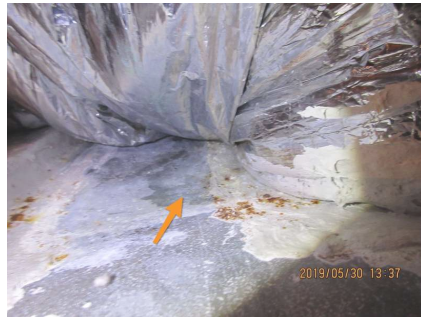
Moisture present on top of AC unit in attic with organic growth. Ductwork should not be laying on anything because it causes condensation which leads to moisture build up.
