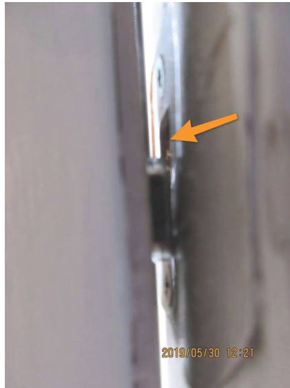
This shows distance that door is off.
