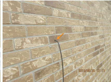
Recommend sealing this to prevent moisture and pest intrusion.
