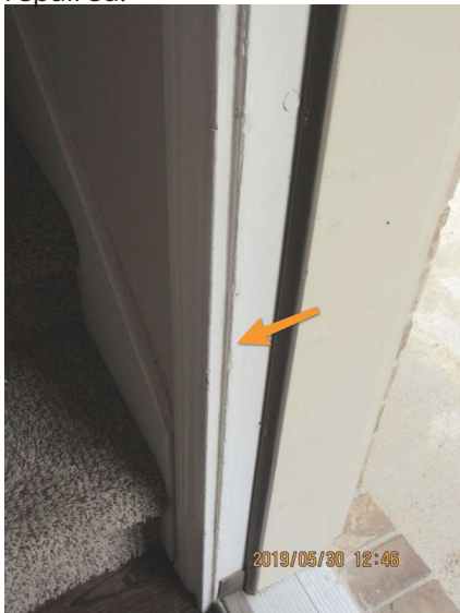
Poor workmanship. Cosmetic only.
