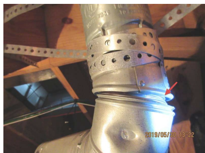
Broken flue.
