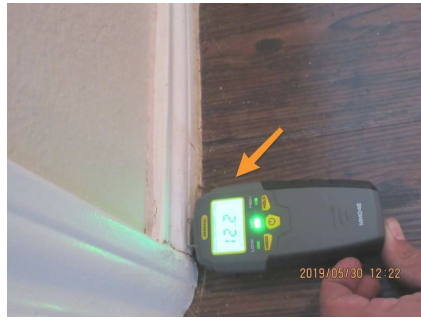
Right side (looking out) of back door. Visible moisture present. This is most likely due to the wood rot around the door not the exterior along with the siding not being 2" above concrete. Recommend removing and seeing what is behind the wood for any further moisture damage.
