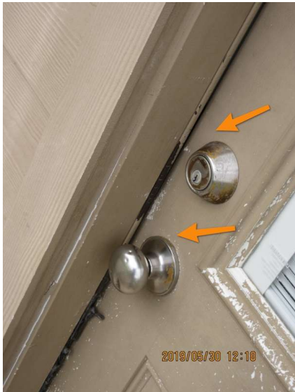
Back door does not close properly. You have to pull up on the door for it too close. Recommend having door repaired.
