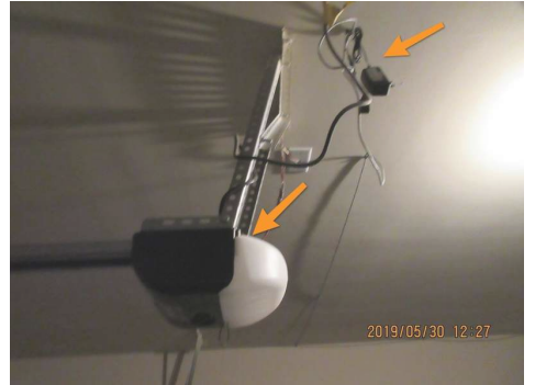
Opener had loud buzzing noise. Recommend removing electrical wiring.
