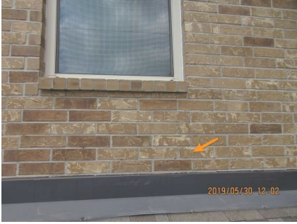
Cracked brick. See comments in "Foundations"
