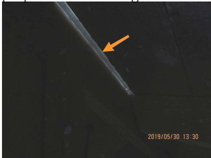
Extent of ridge vent.
