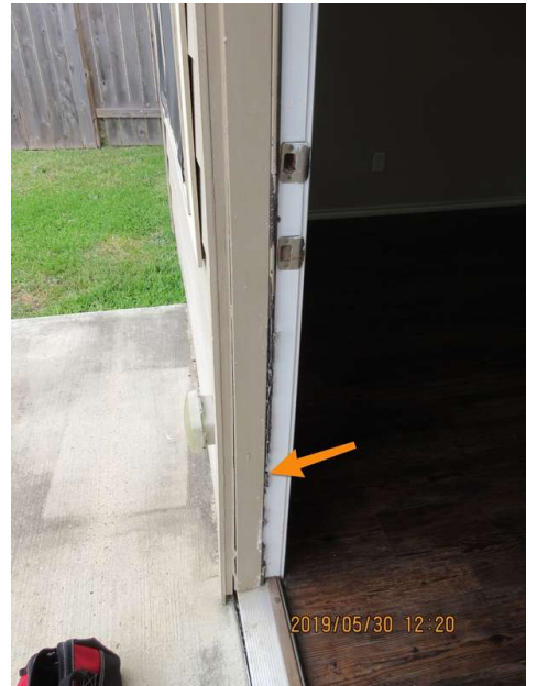
Weather stripping is damaged. Recommend replacing for proper sealing of house.
