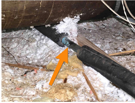
Condensation Inside Attic
