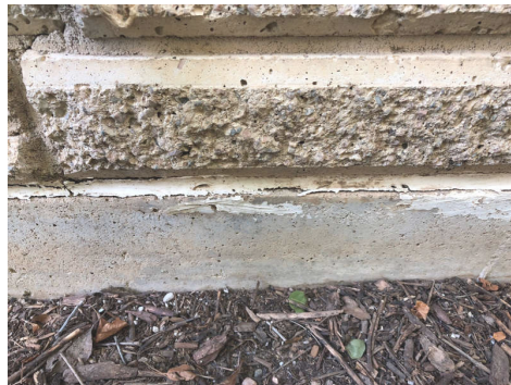
1st Floor West
