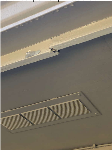
1st Floor West Exterior
