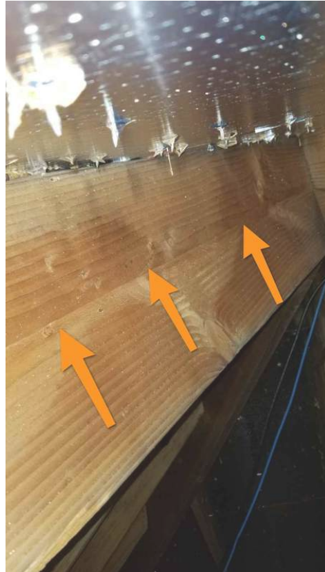
Above Garage Attic Hatch
