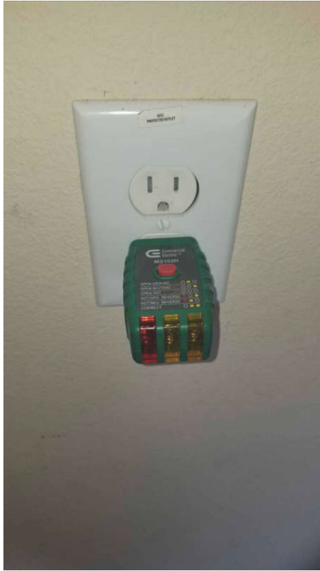
Garage Near Door
