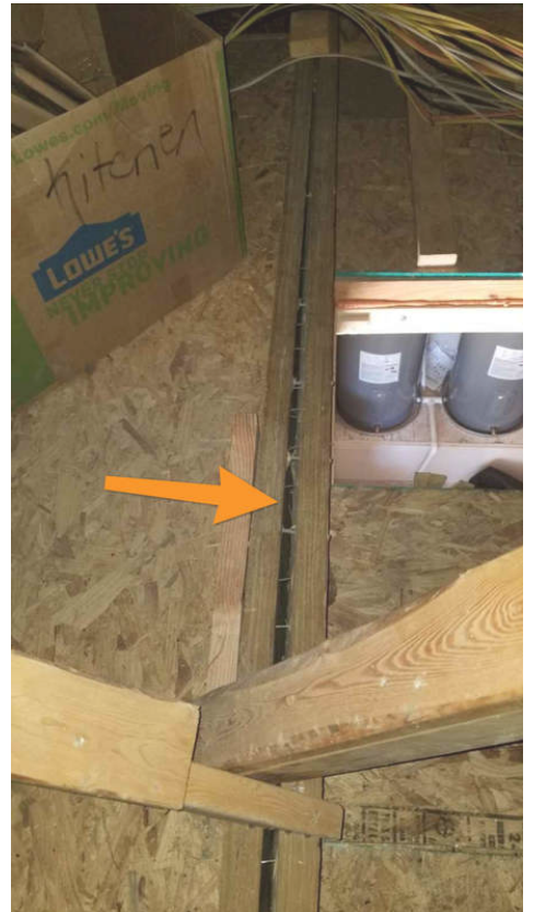
Attic Above Garage
