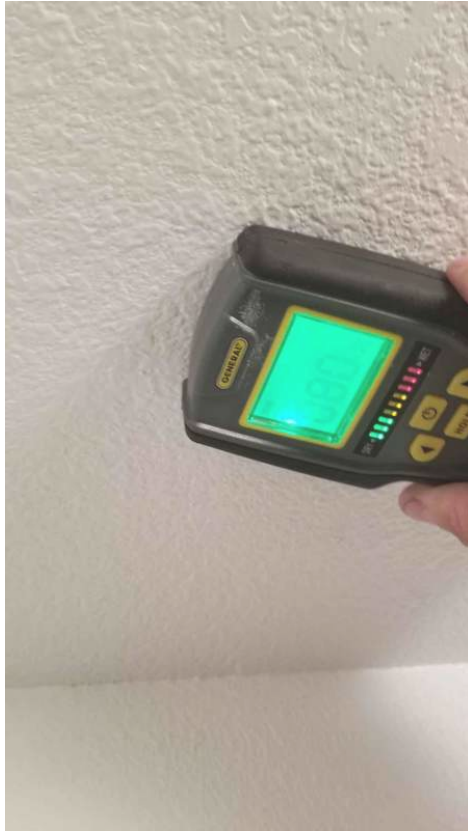
High Moisture, 2nd Floor Closet Ceiling
