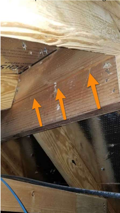
Above Garage Attic Hatch
