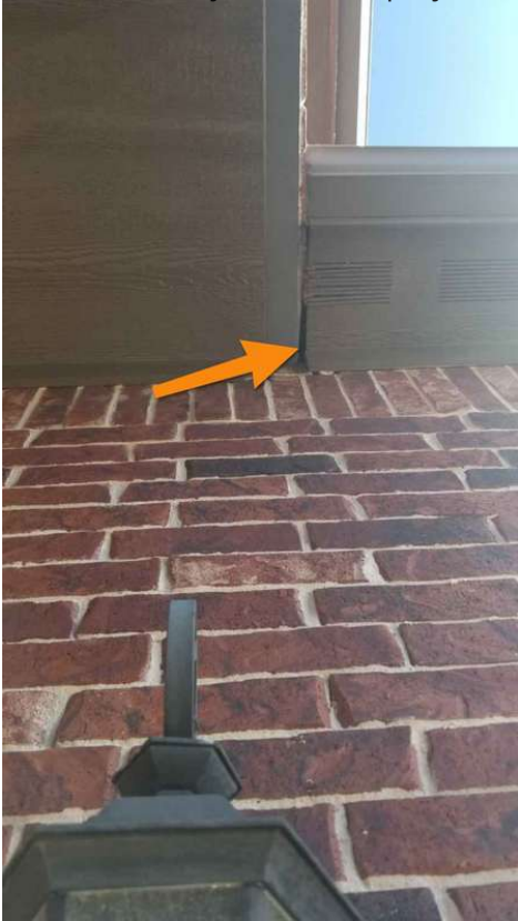
Above Front Porch, Exterior View
