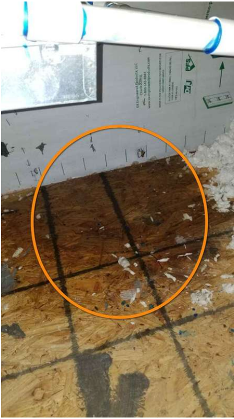
Area of Moisture
