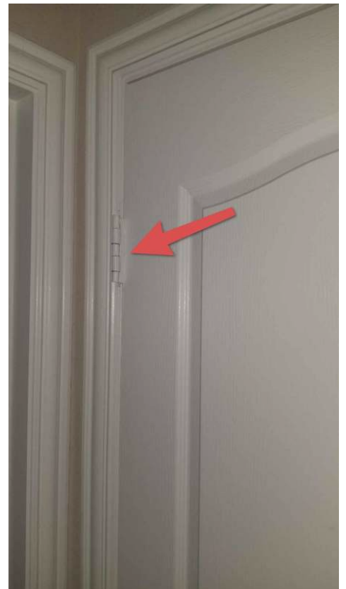
Door Leading to Garage Needs Self-closing Hinge
