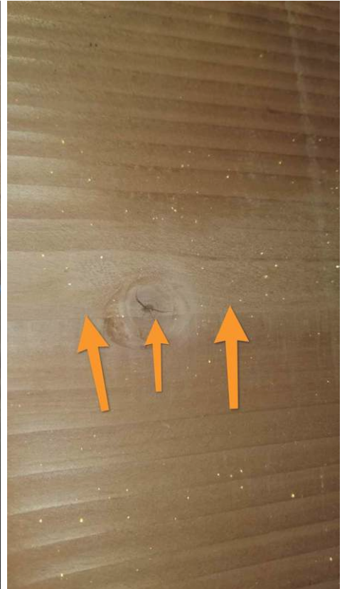
Above Garage Attic Hatch
