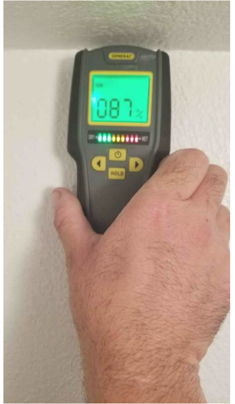
High Moisture Level , 2nd Floor Closet Wall
