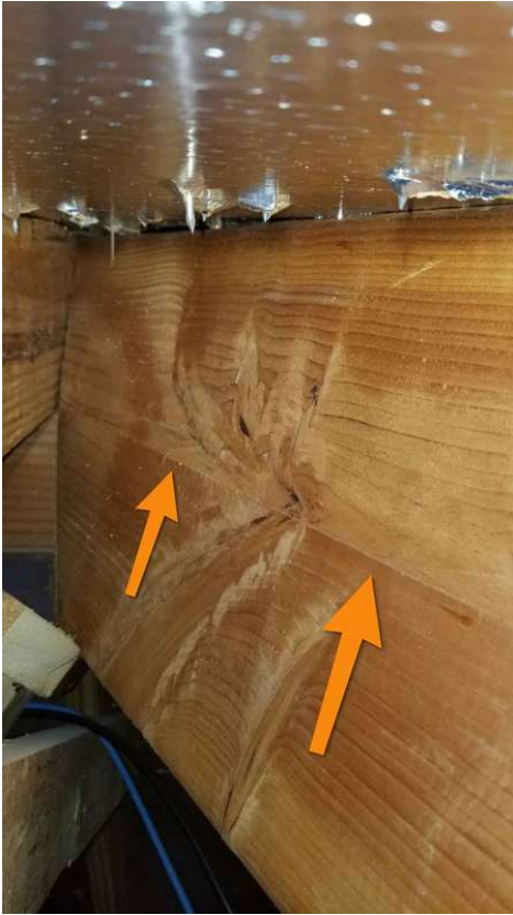
Above Garage Attic Hatch
