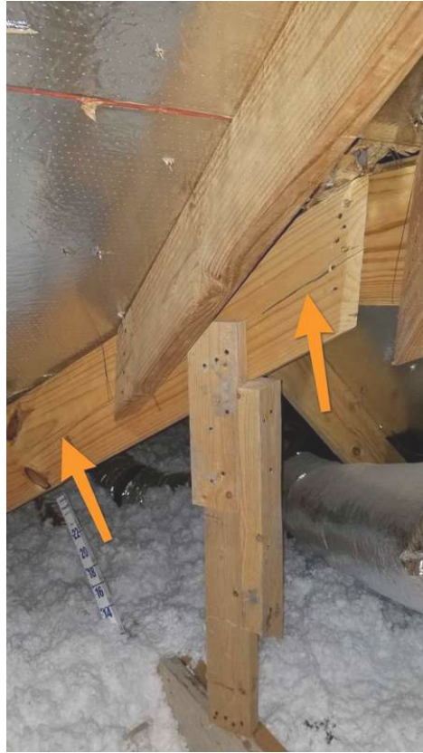
Attic Above Master Bedroom
