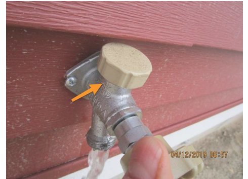
Leak observed at hose bib
