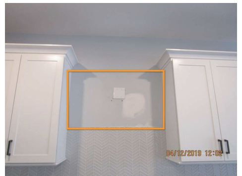
Kitchen-Exhaust hood missing
