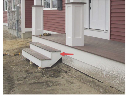
Steps were removed during inspection. Front Steps
