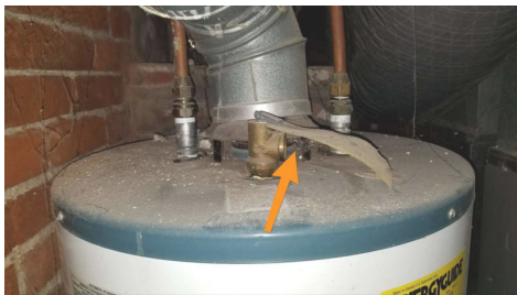
DISCHARGE PIPE ON TPR VALVE
