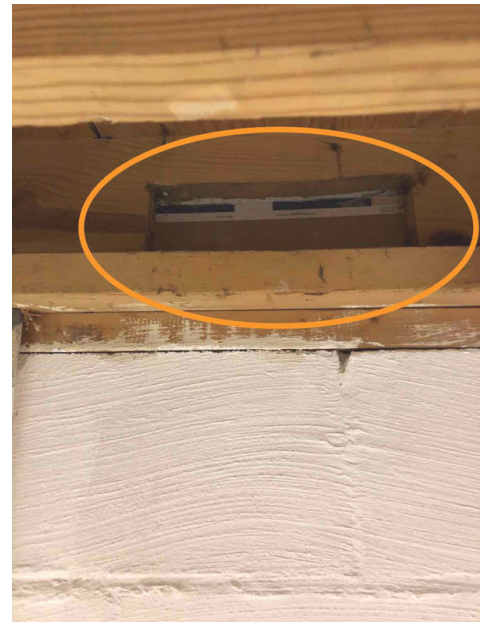
Northwest work room North wall
