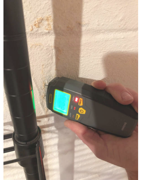
Northeast storage room
