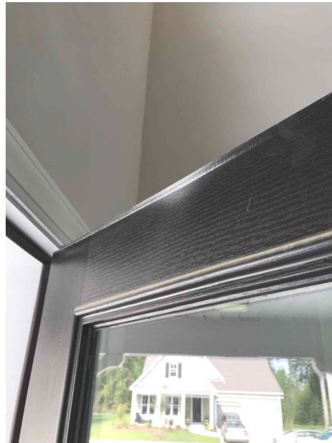
Front door had paint on it
