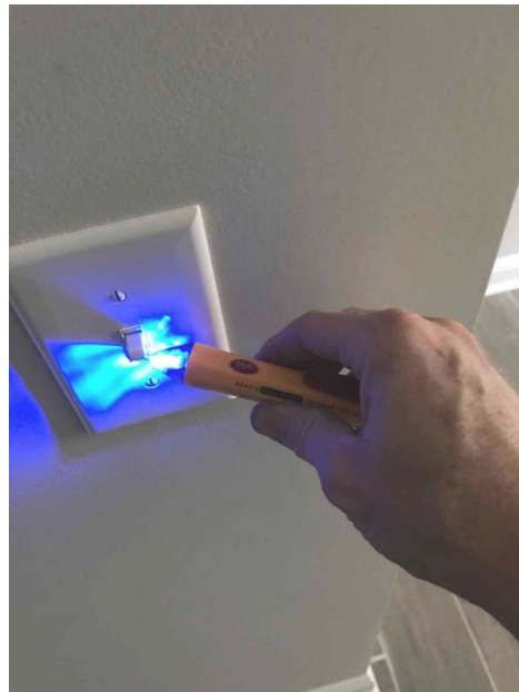
Switches are not hot
