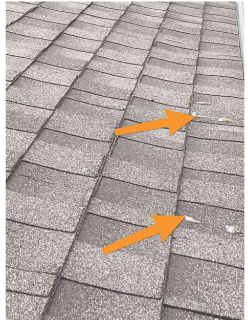
Silicone sealant covered nails through shingle tabs from installation
