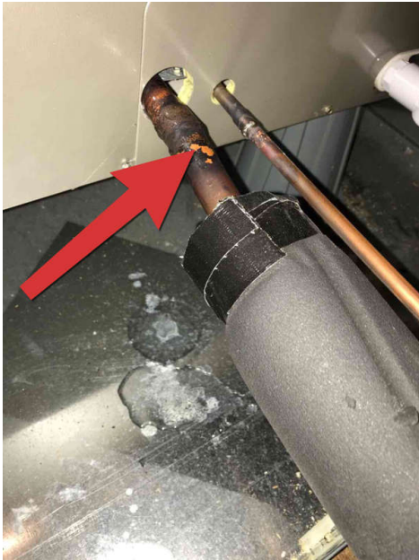
Water in pan from leaking copper Piping
