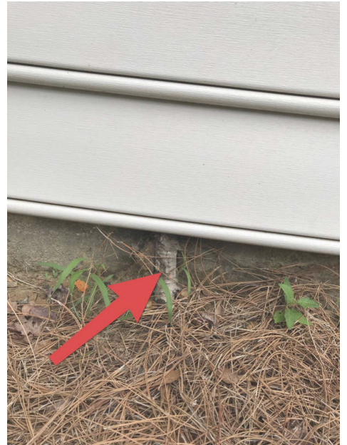
Tree growing under siding
