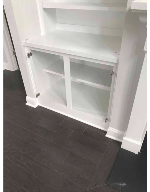
Cabinet Door are Missing in Living Room
