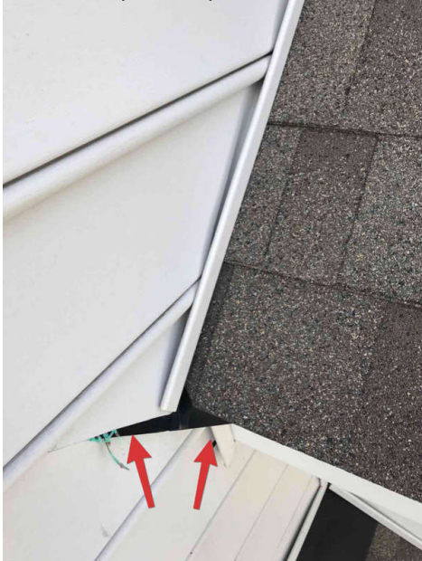
Cut in siding
