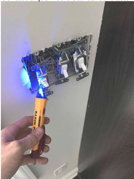
Cover needs to be placed over switches and they were not hot at the time of the inspection.
