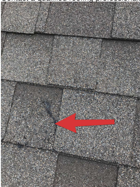
Crack shingle on right elevation towards front of home
