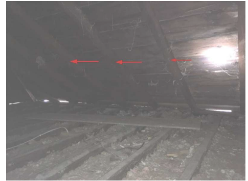
Kneewall supports may be required to support roof and snow loading
