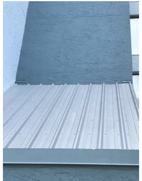
South, Missing Headwall Flashing
