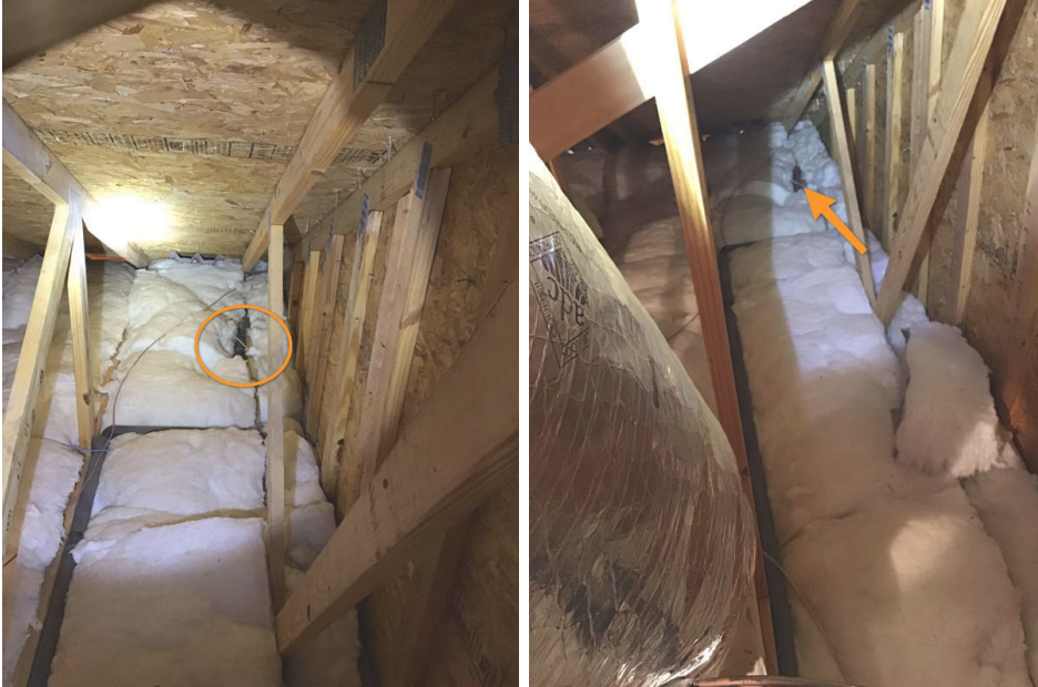
Area is behind the air handler in the corner of the attic.
