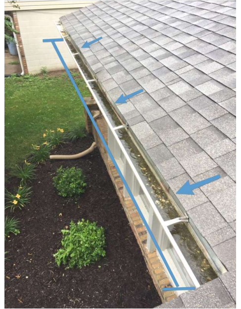
Approximately two inches of standing water in gutter.
