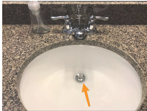
Master Bathroom Sink #1
