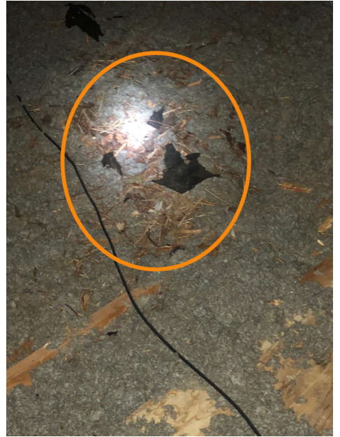
Attic near access
