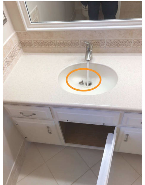
2nd Floor hall Bathroom
