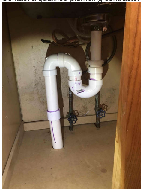
S-Trap vs. P-Trap
