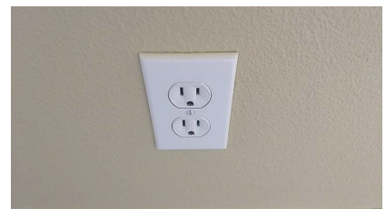
2nd Floor Hallway
