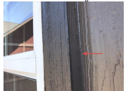
West - Needs resealing
