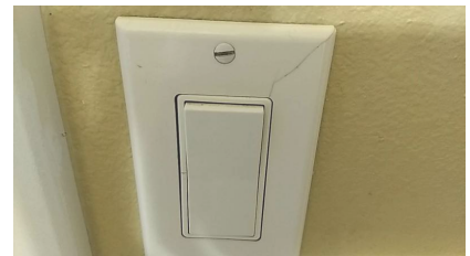
2nd Floor Bathroom
