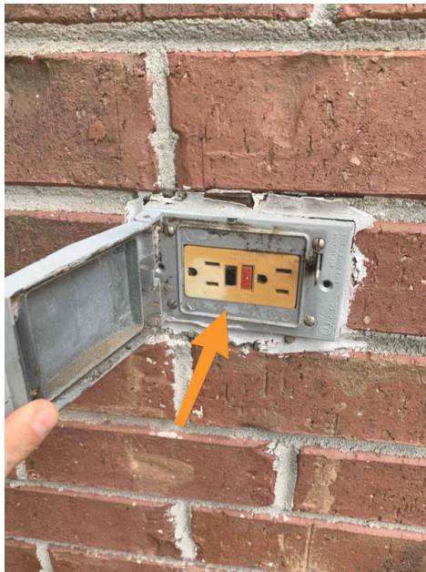
Front of the home, left of front steps
