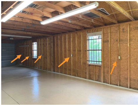
ALL receptacles in the detached garage
