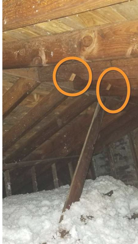
Notches cut out of rafters
