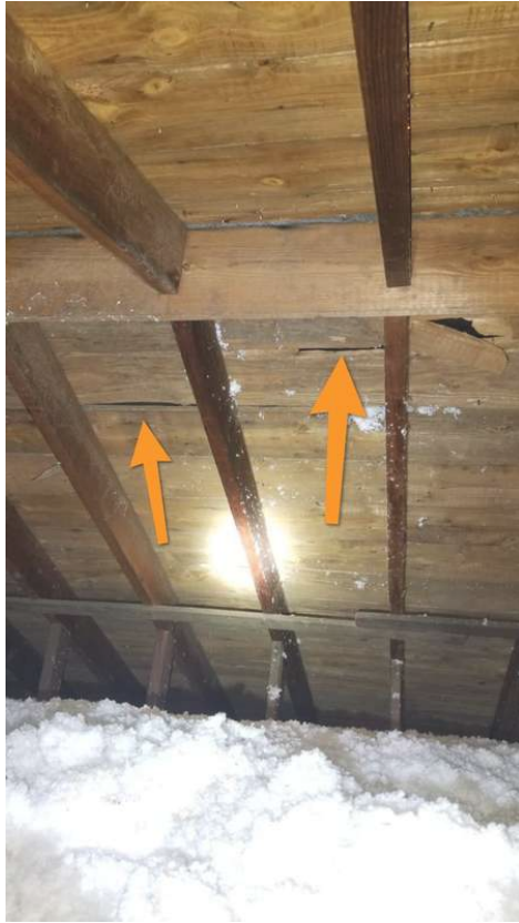
Planks are showing splitting and signs of separation occurring. Recommend a roofing professional to further evaluate
