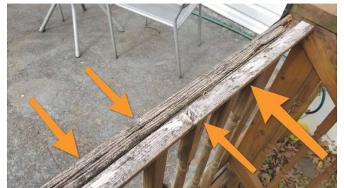
Deck gate top rail
