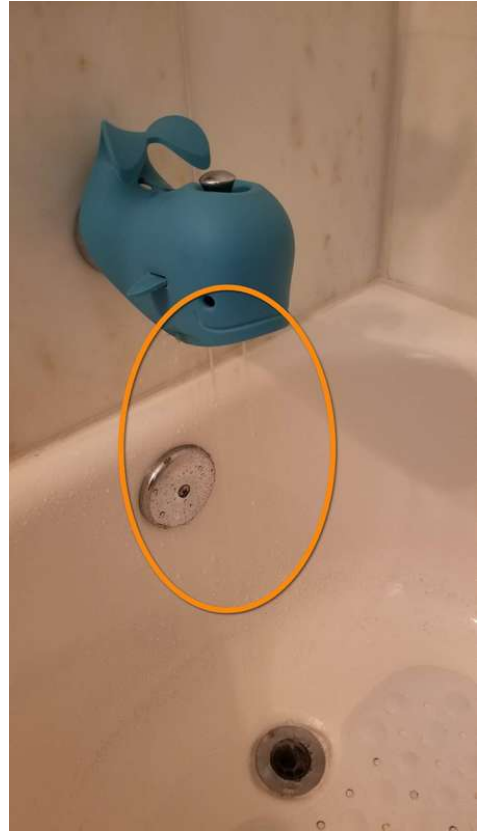
Water not properly diverting to the shower head
