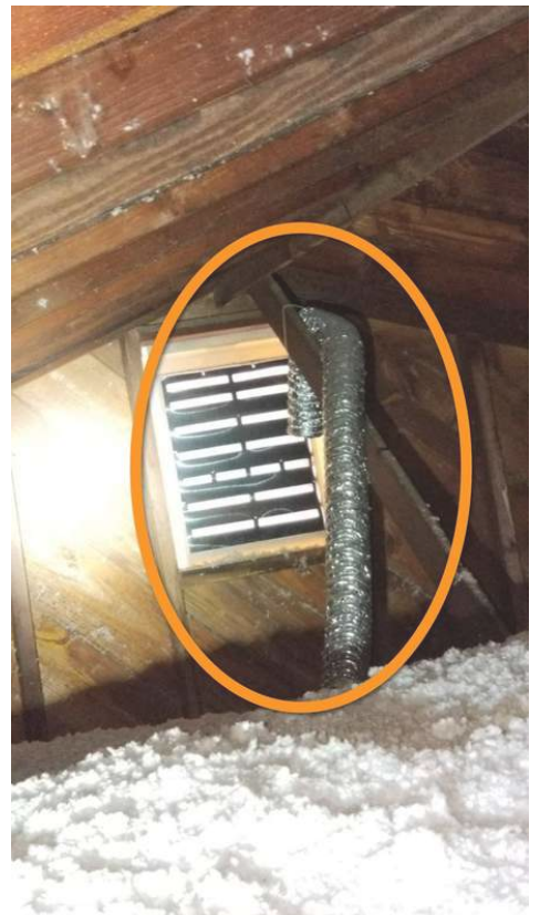
Vent hose appears to discharge into the attic. Proper venting is needed to discharge out of the attic and to the exterior of the house
