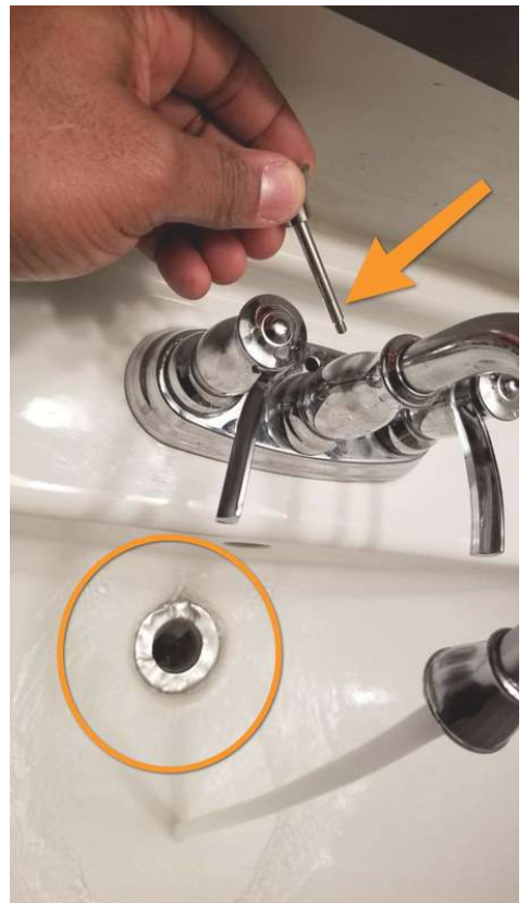
Stopper missing and broken
