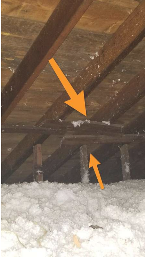
Improper bracing of rafters with wood not deemed suitable
