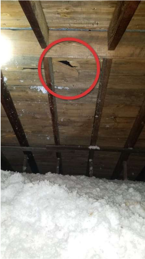
Large hole from broken roof plank covered with underlayment and shingles
