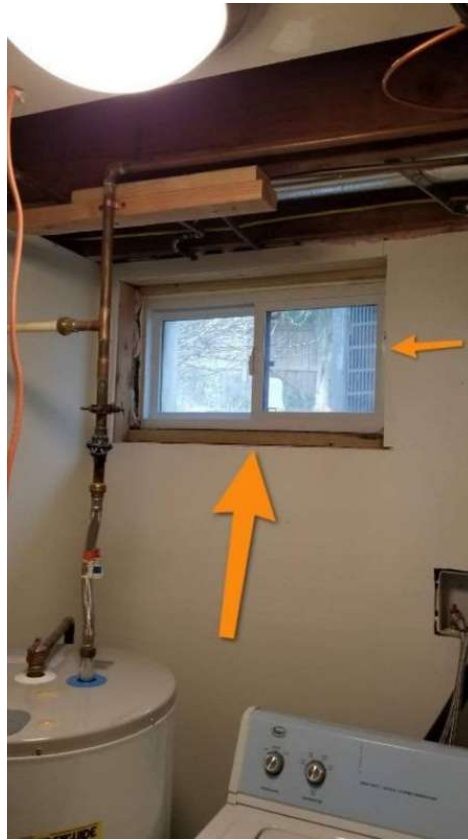
Laundry room window. Not an egress window
