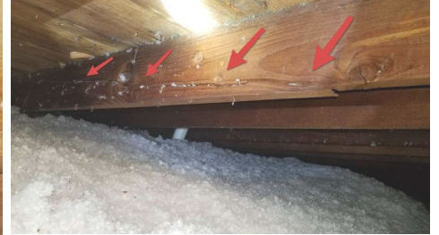
Rafter is splitting very badly and needs to be evaluated by a roofing professional
