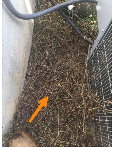
Rear of a/c unit
