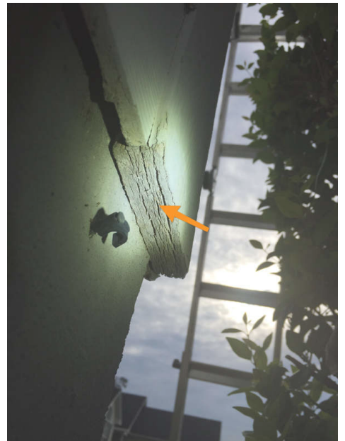
Engineered wood coming apart at ends
