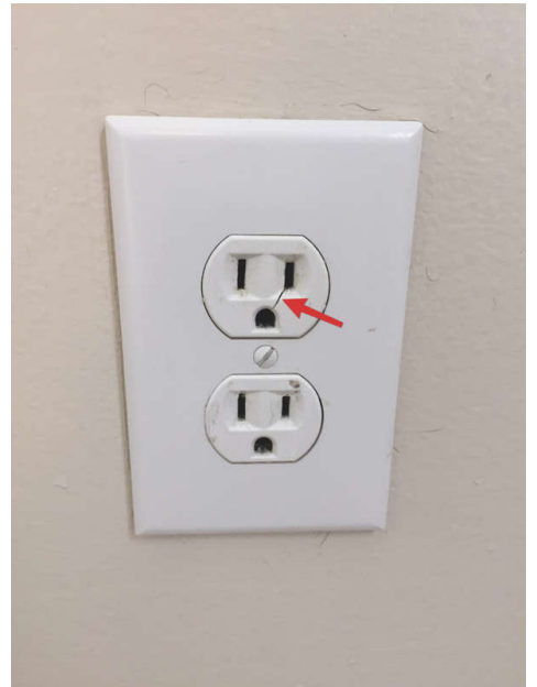
Crack may get worse with use
