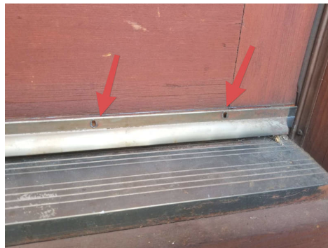
Missing screws
