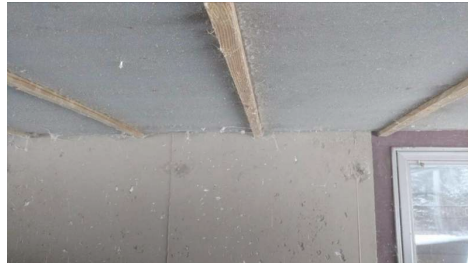
Underneath the back porch, when viewed with a flashlight the ledger was visible, but not able to be photographed.
