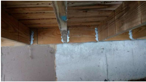
Underneath the front porch.
