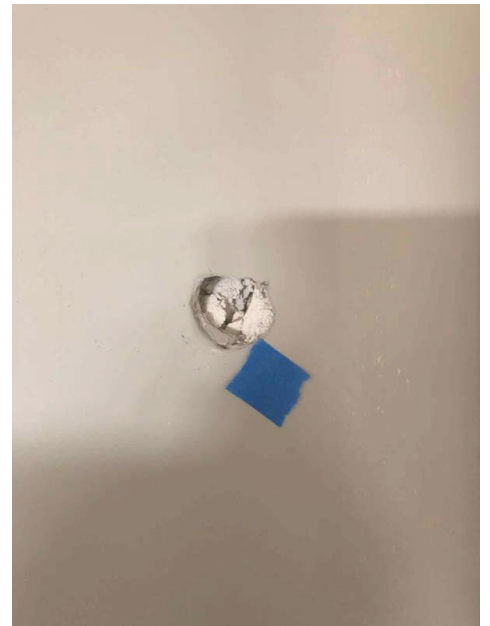
Garage East Wall
