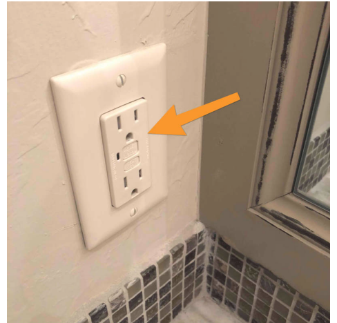
1st Floor 1/2 Bathroom
