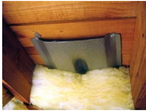
Properly Installed Insulation Baffles
